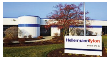
Offices and Manufacturing 87th Street, Milwaukee, WI
