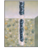
Doweling into Concrete with Rebar
