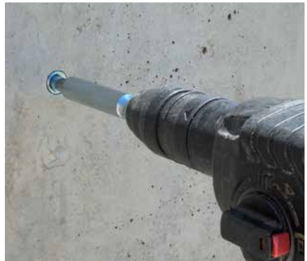
Anchor being set with SDS setting tool.
